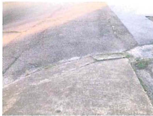
Post Oak Ave – A perpendicular ramp is present on one side with no detectable warning surface and no curb cut on the other. No crosswalk is present.
