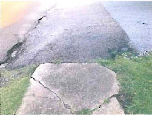
Robin Ave – Perpendicular ramp with no detectable warning surface on one side and no curb cut on the other. No crosswalk is present. Also, note the heavy damage.
