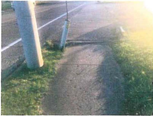
Cole Ave – Perpendicular ramp is present with no warning surface. No crosswalk is present.
