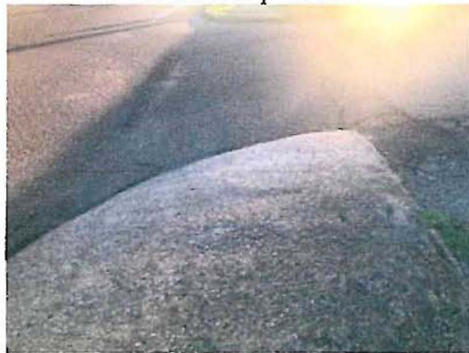
Post Oak Ave – A perpendicular ramp is present on one side with no detectable warning surface and no curb cut on the other. No crosswalk is present.
