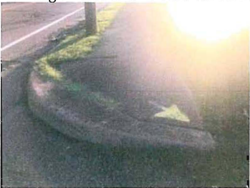
Post Oak Ave – A perpendicular ramp is present on one side with no detectable warning surface and no curb cut on the other. No crosswalk is present.
