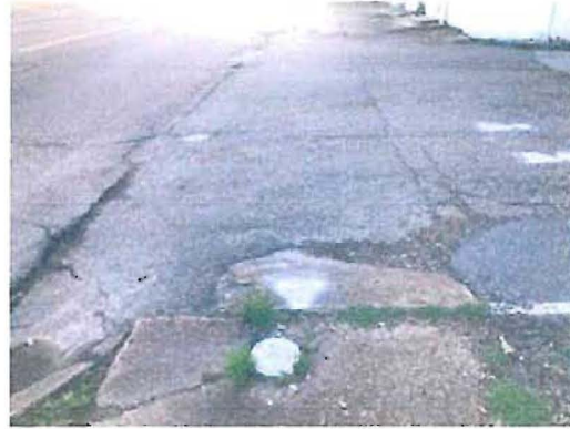
Robin Ave – Perpendicular ramp with no detectable warning surface on one side and no curb cut on the other. No crosswalk is present. Also, note the heavy damage.
