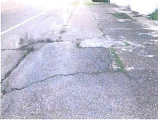
Robin Ave – Perpendicular ramp with no detectable warning surface on one side and no curb cut on the other. No crosswalk is present. Also, note the heavy damage.
