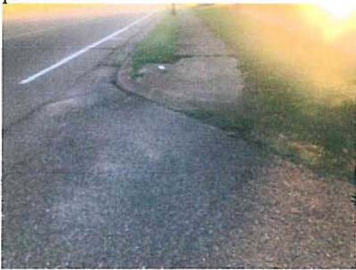
Post Oak Ave – A perpendicular ramp is present on one side with no detectable warning surface and no curb cut on the other. No crosswalk is present.
