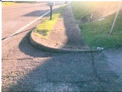
Washington Ave – Diagonal ramp on one side with no detectable warning surface and no curb cut on the other. No crosswalk is present.
