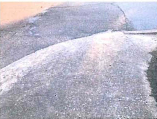
Washington Ave – Diagonal ramp on one side with no detectable warning surface and no curb cut on the other. No crosswalk is present.
