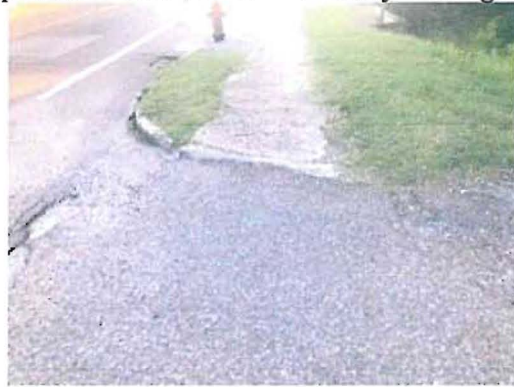
Robin Ave – Perpendicular ramp with no detectable warning surface on one side and no curb cut on the other. No crosswalk is present. Also, note the heavy damage.
